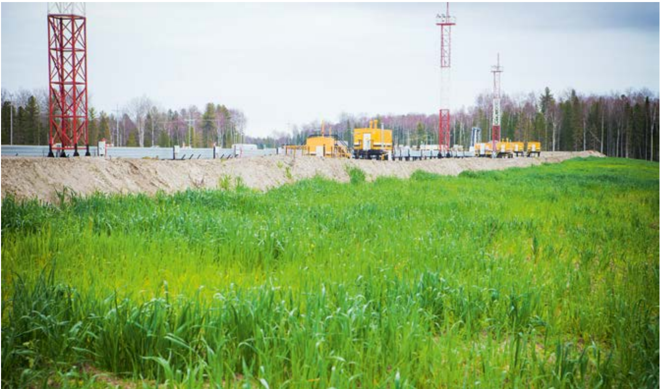
Remediated legacy sludge pit, LLC RN-Yuganskneftegaz
