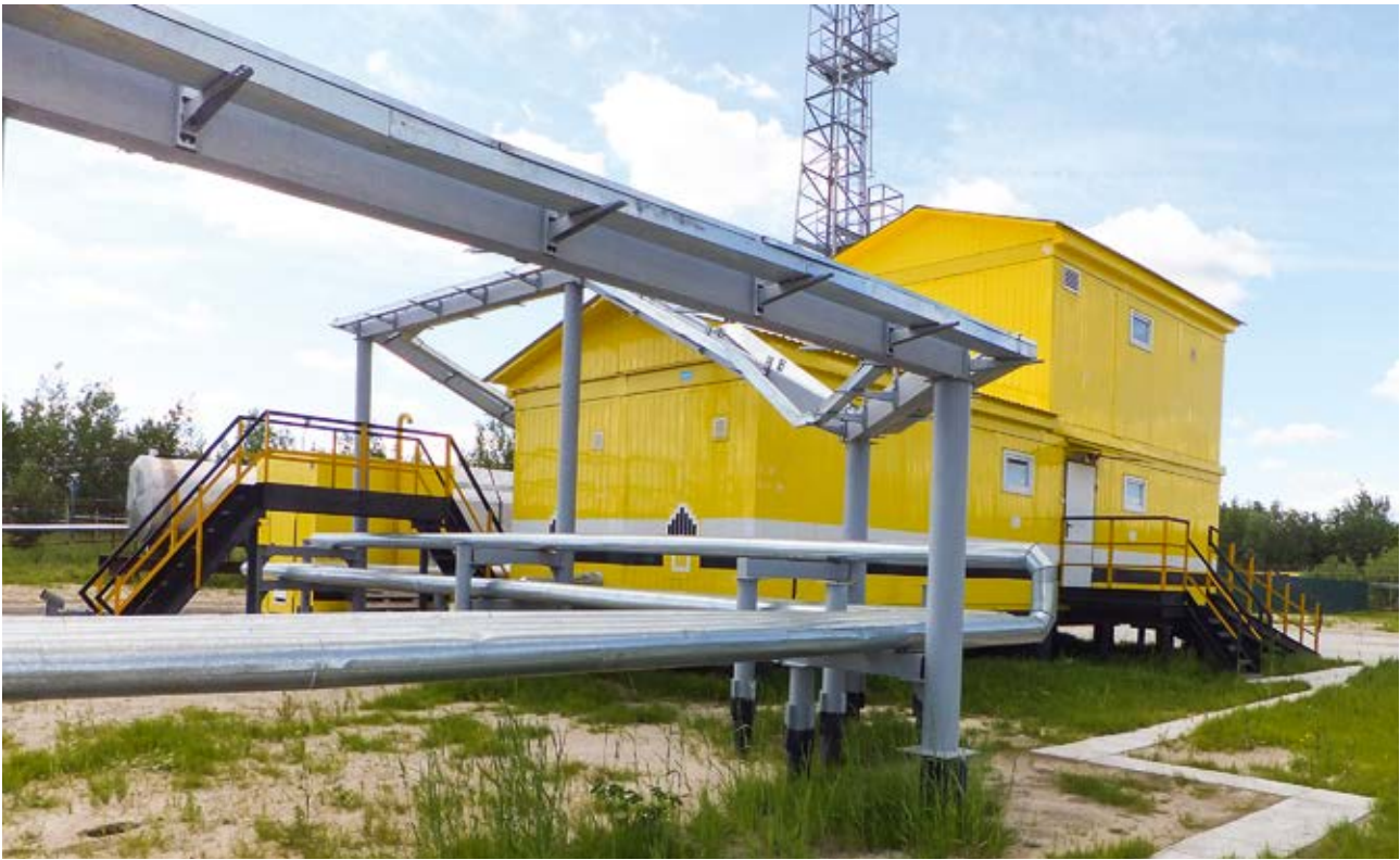
Well clean up unit, LLC RN-Yuganskneftegaz
